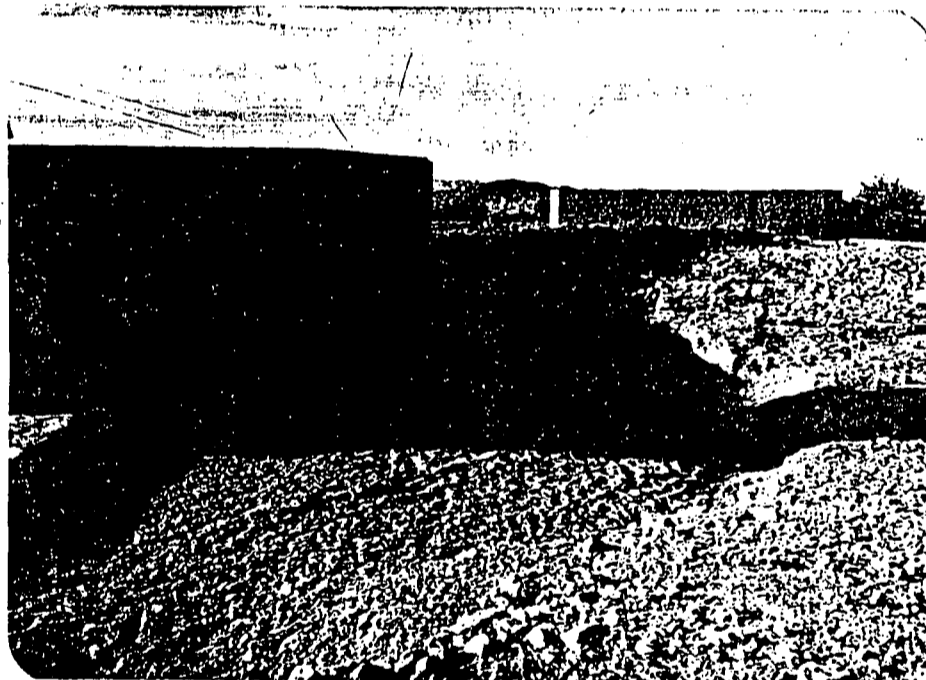
Photo-3.5 Rakhni Irrigation Scheme-Balochistan. Crest of extension weir one meter higher than original weir.
